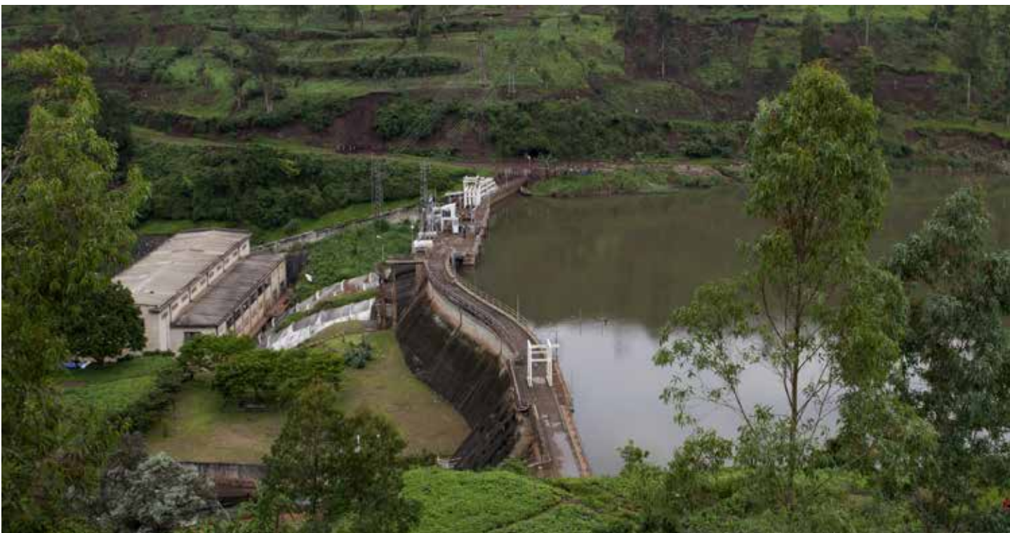
The Ruzizi I hydropower plant on the Ruzizi River, bordering Rwanda and DR Congo
