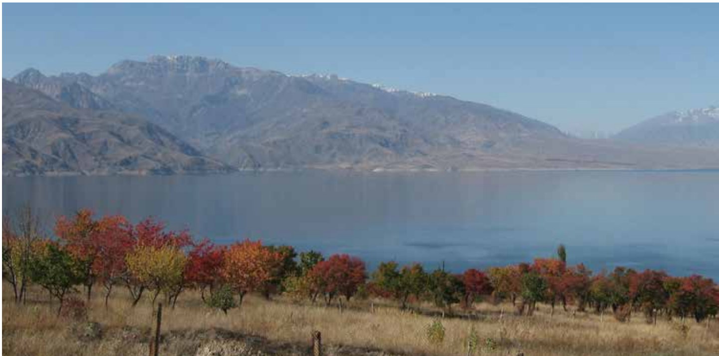
The reservoir at the 1,200 MW Toktogul hydro project on the Naryn River (Kyrgyzstan), which is currently undergoing rehabilitation and upgrade
